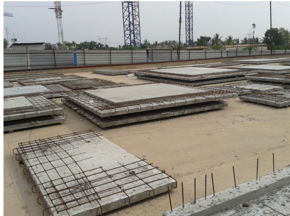
SLAB PANELS STACKING
