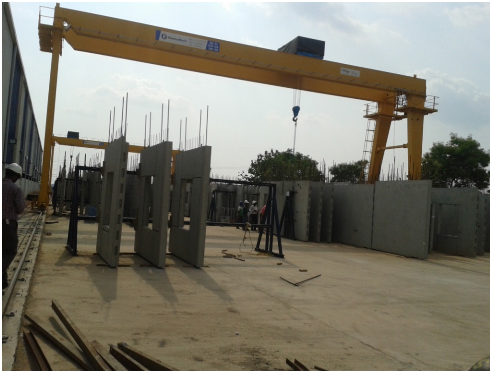
WALL PANELS STACKING
